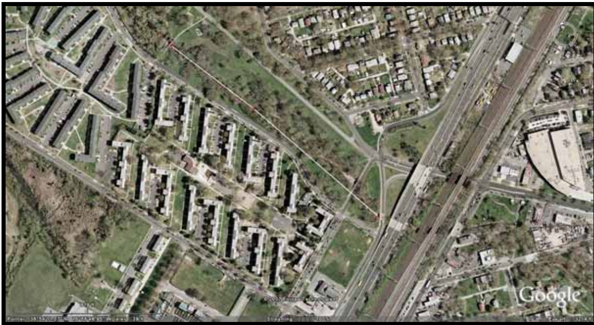
Figure 3.1.25 Watts Branch: Kenilworth Ave – Foot Bridge
