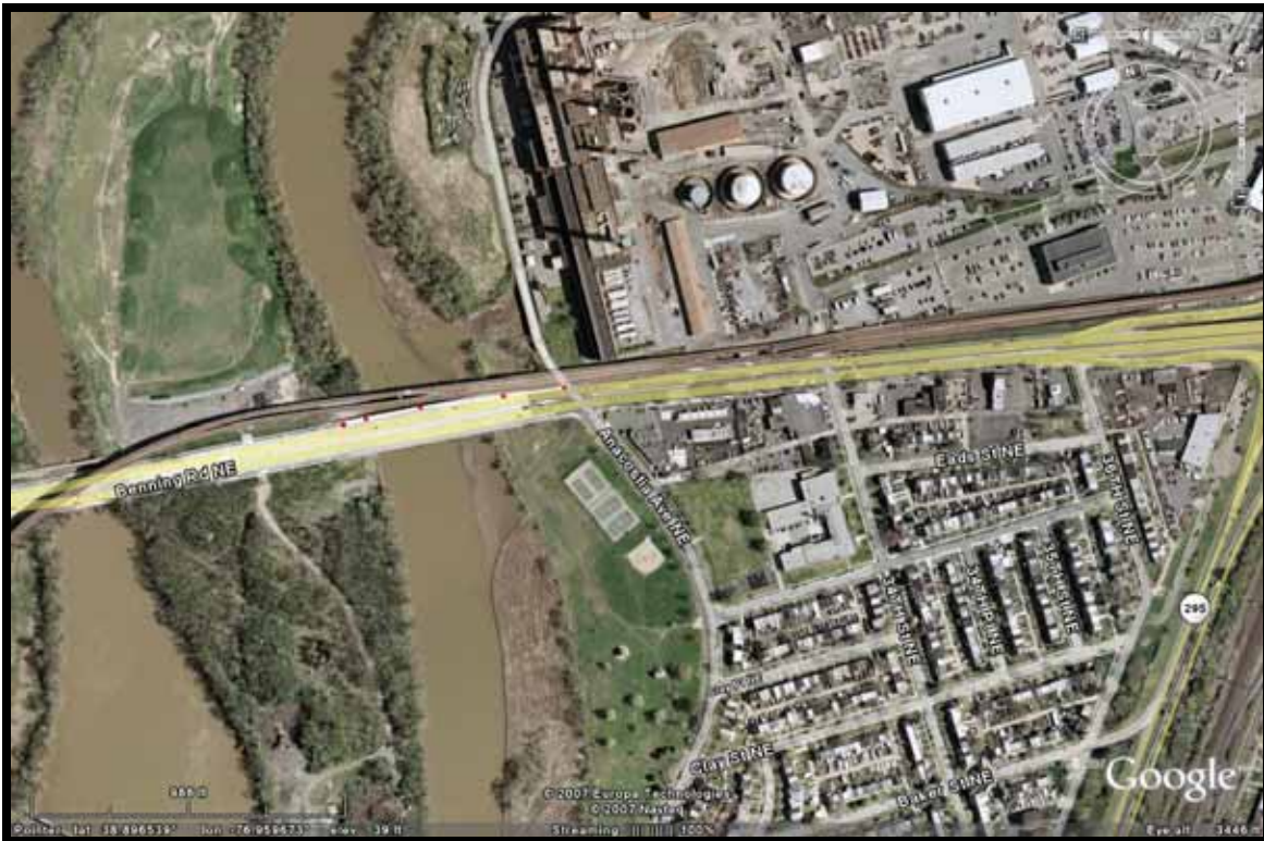
Figure 3.1.65 Benning Road Northbound
