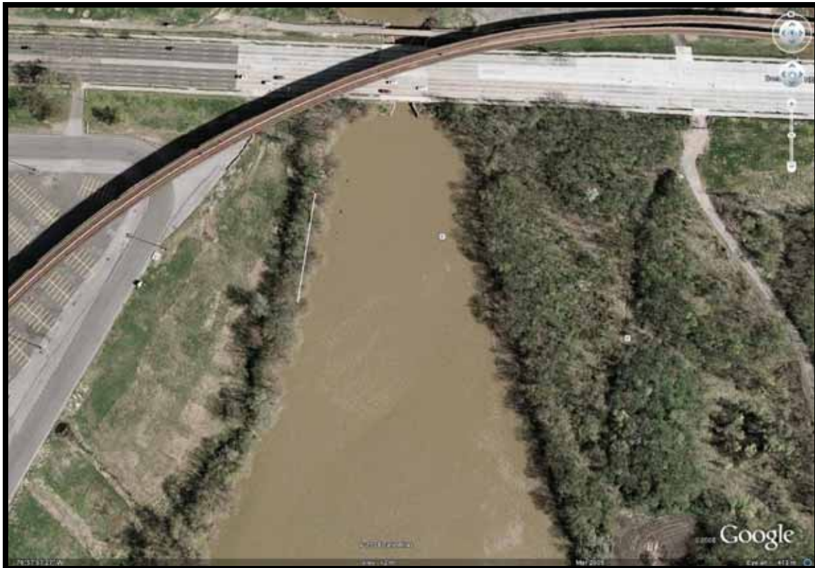
Figure 3.1.11 Kingman Lake: Benning Road Bridge Downstream
