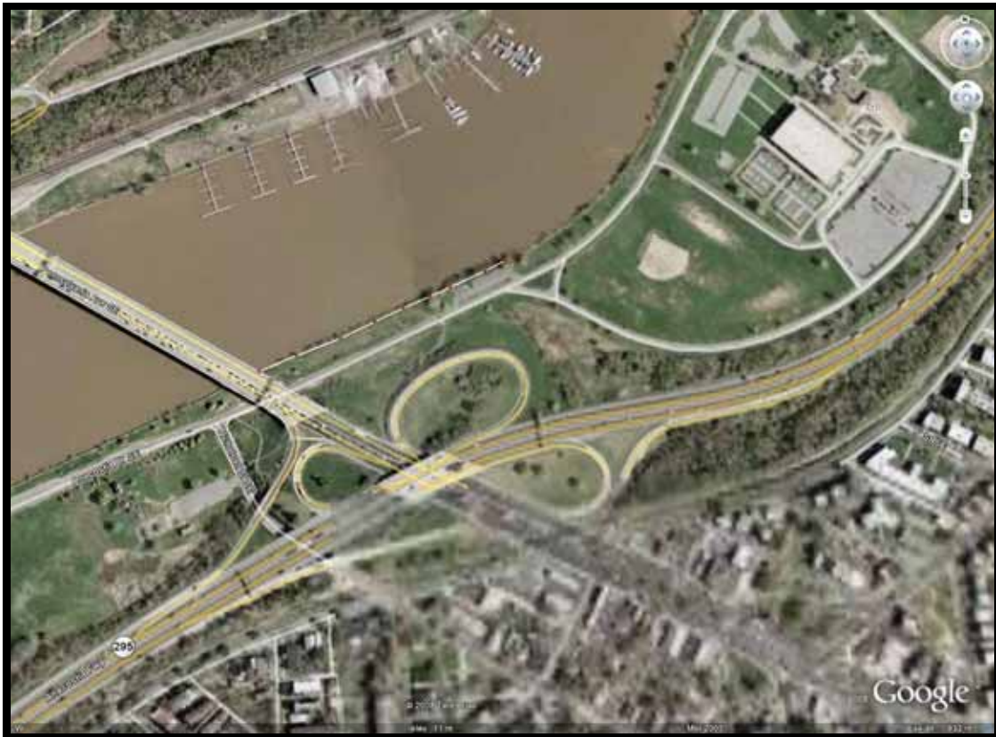
Figure 3.1.6 Anacostia: Pennsylvania Avenue Storm Sewer
