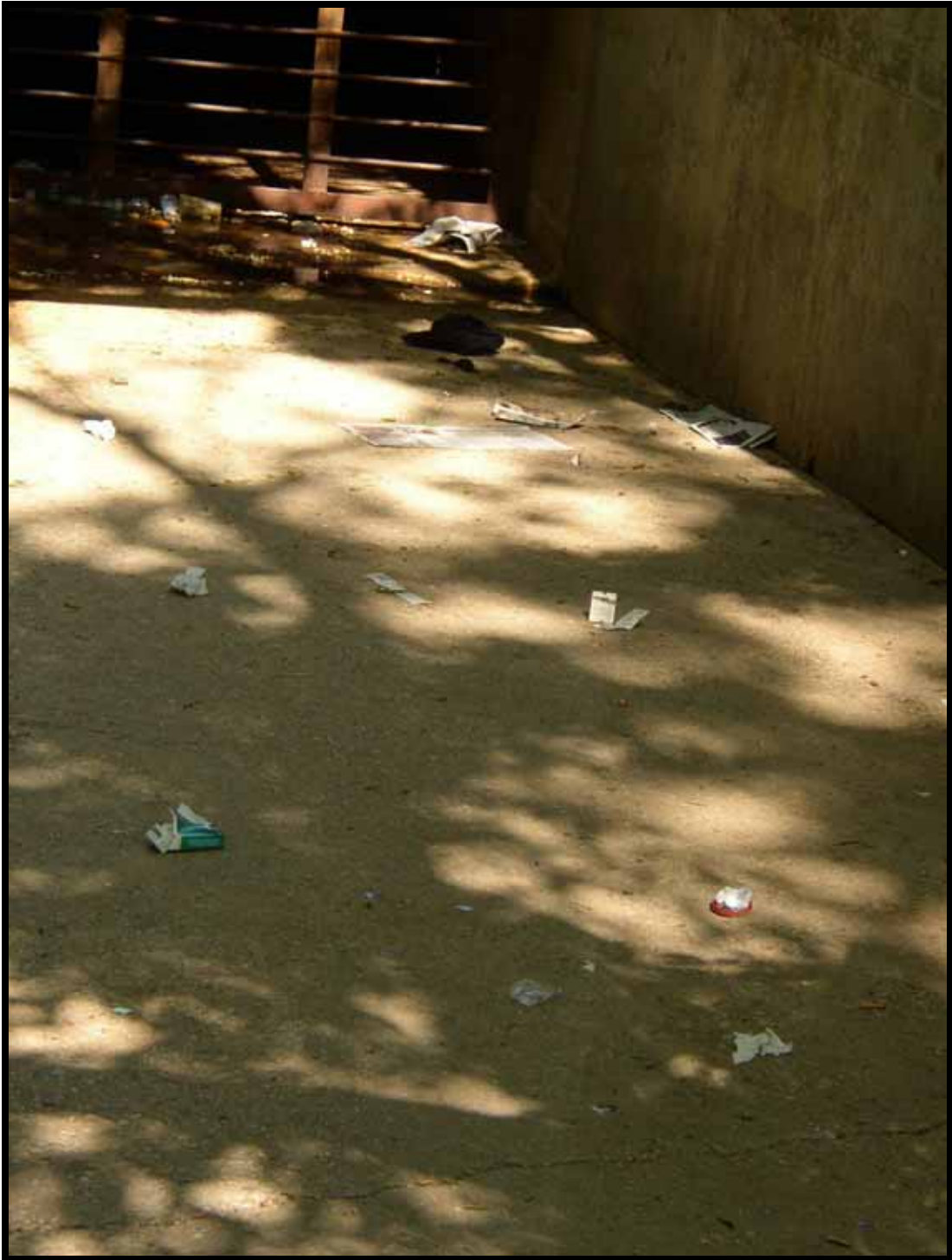
Figure 3.2.37 Trash found in the streambed
