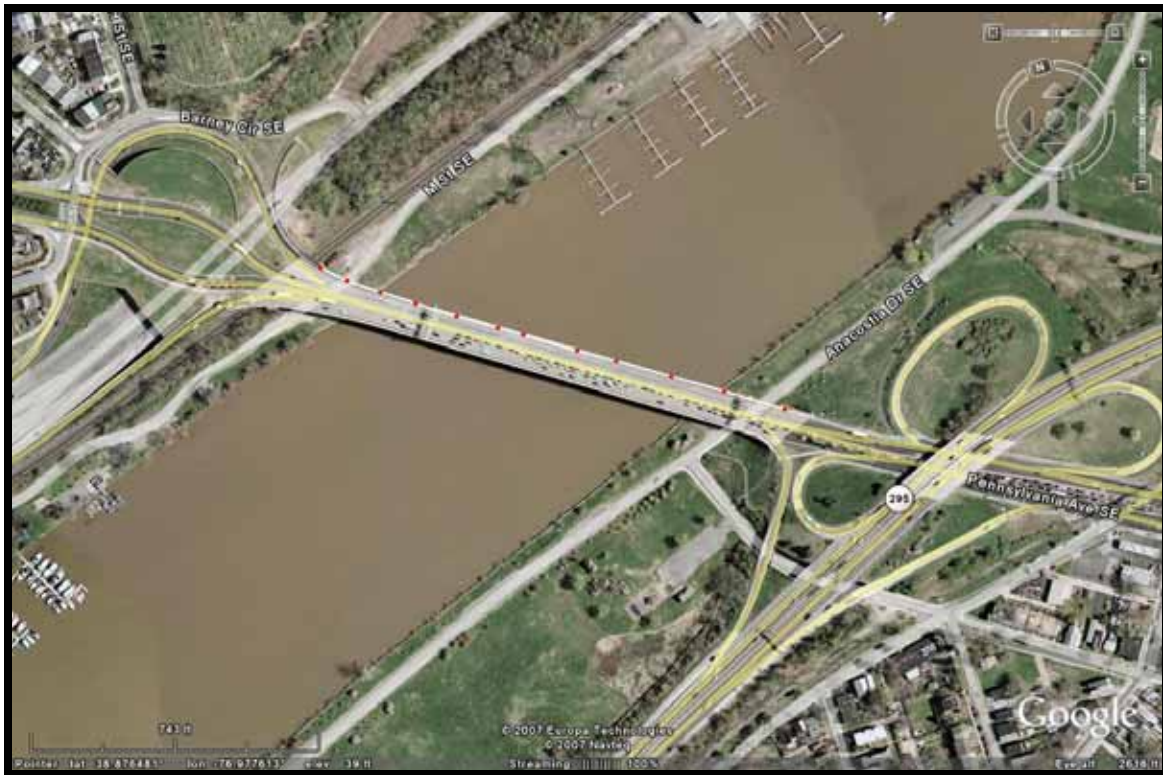
Figure 3.1.64 Penn Ave Northbound
