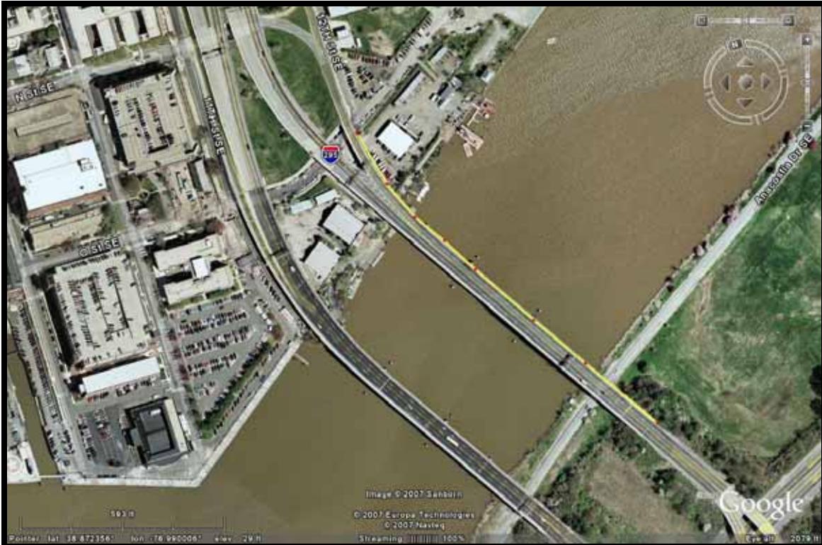
Figure 3.1.66 11 th Street Bridge Northbound
