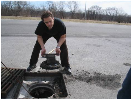
A catch basin insert with collected pollutants
