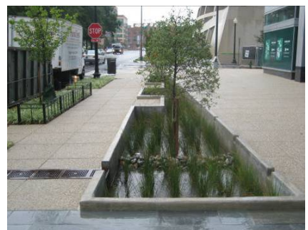
Roadway pollutants being captured in a bioretention cell
