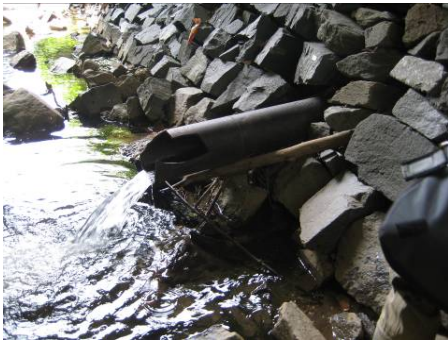
An outfall discharging during dry weather
