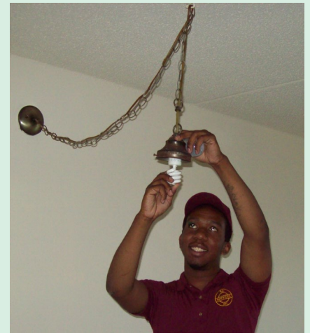
Installing CFLs at Vicksburg Senior Village
