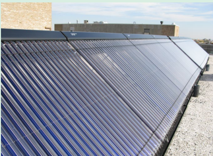
Solar hot water collectors at American University
