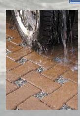
Pervious Pavement prevents stormwater runoff by allowing water to drain through or around the pavement into the ground.
